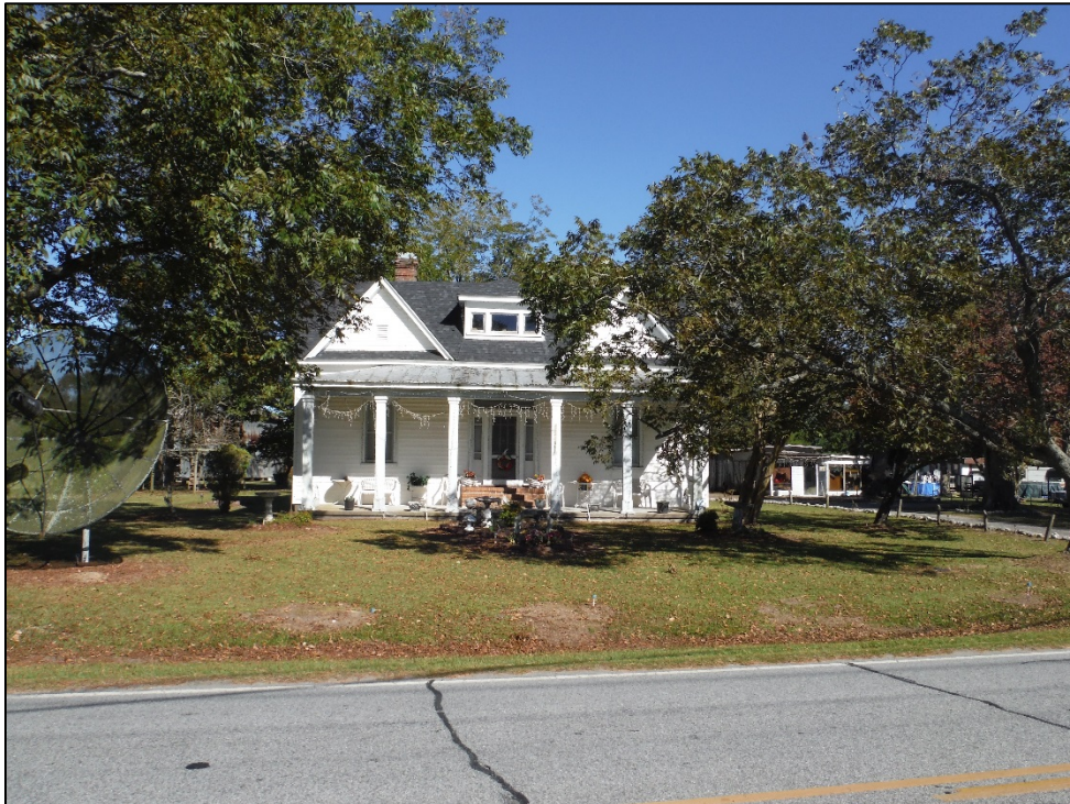
Figure 11. View of Enzel Sullivan House (LR0889) (PIN 450601467006) from Hull Road, facing northeast.
