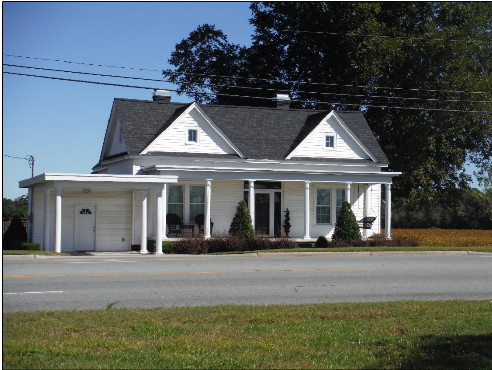
Figure 3. View of the Poole-Smith House (LR0883) (PIN 450601377762) from Highway 258 N, facing east.
