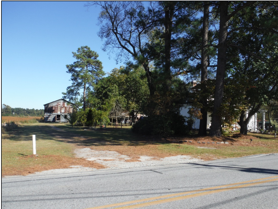
Figure 14. View of Enzel Sullivan House (LR0889) outbuildings from Hull Road, facing east.
