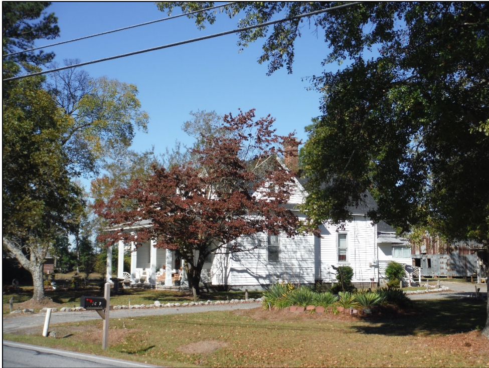
Figure 12. View of Enzel Sullivan House (LR0889) (PIN 450601467006) from Hull Road, facing north.
