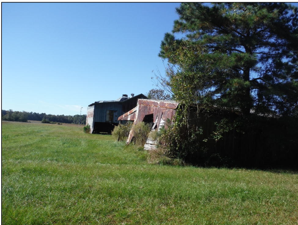
Figure 23. View of Rouse House and Outbuildings (LR1599), barns, facing west.
