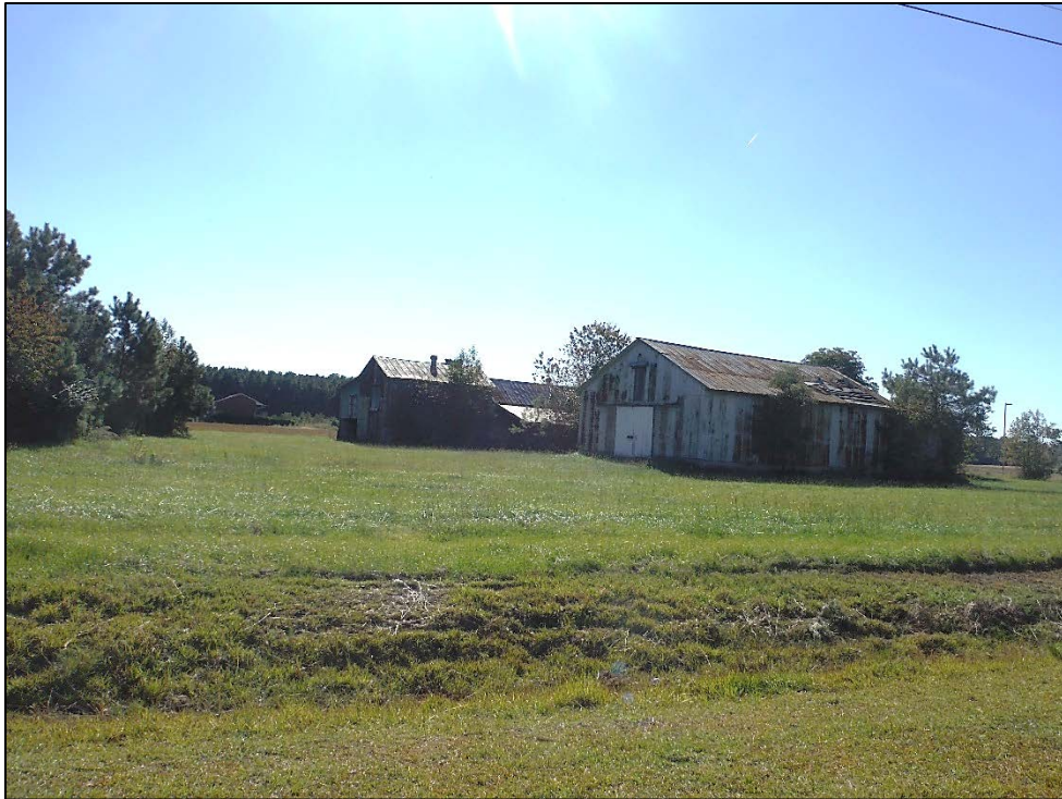
Figure 22. View of Rouse House and Outbuildings (LR1599), barns, facing southwest.
