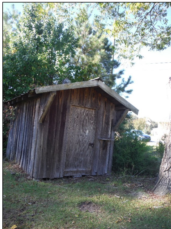
Figure 27. View of Rouse House and Outbuildings (LR1599), outhouse, facing west.
