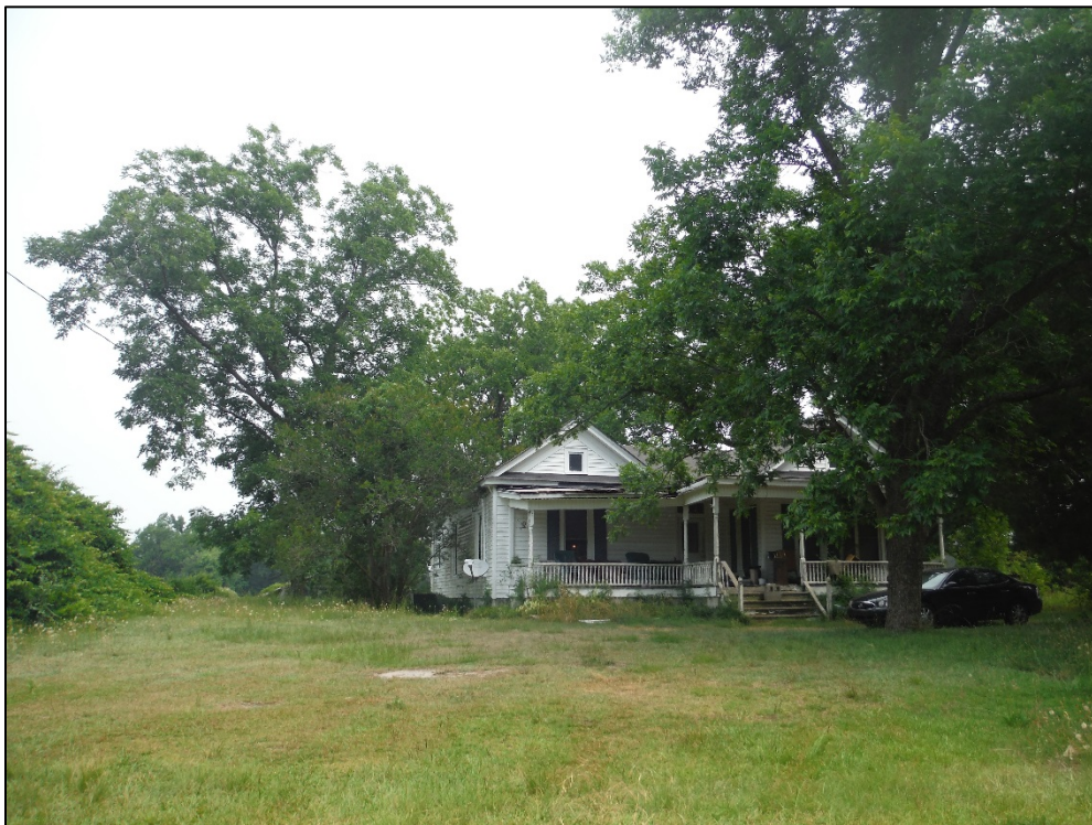
Figure 7. Photo of the Felix Hills House (LR0746), facing northwest.
