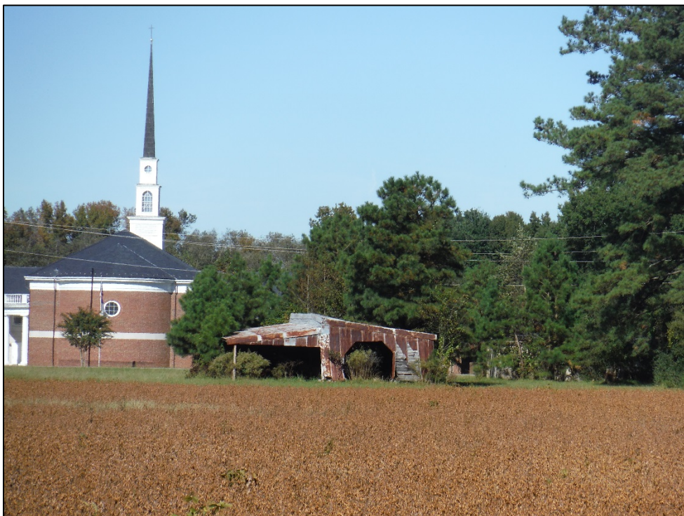
Figure 25. View of Rouse House and Outbuildings (LR1599), tobacco barn, facing northeast.
