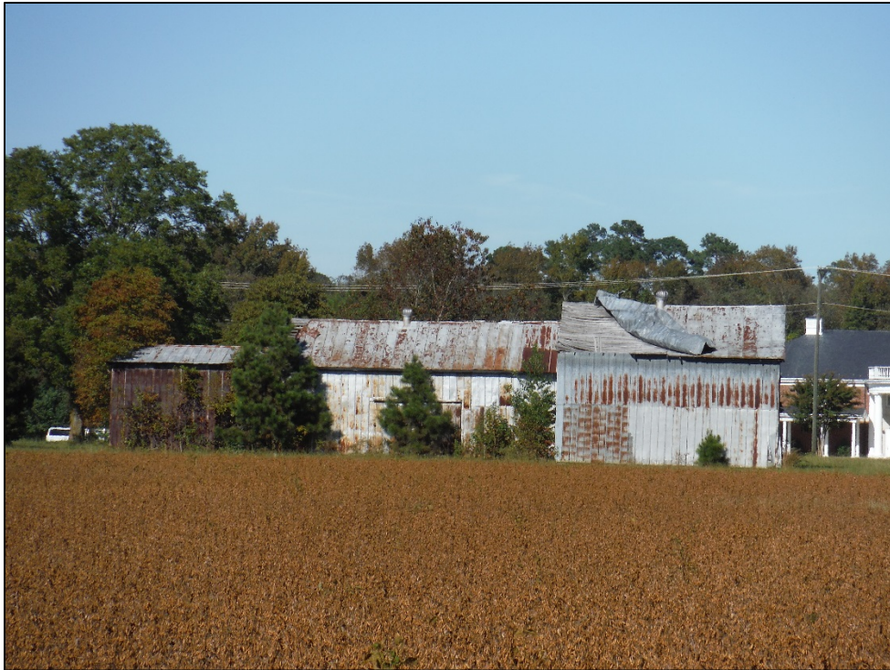
Figure 24. View of Rouse House and Outbuildings (LR1599), barns, facing north.
